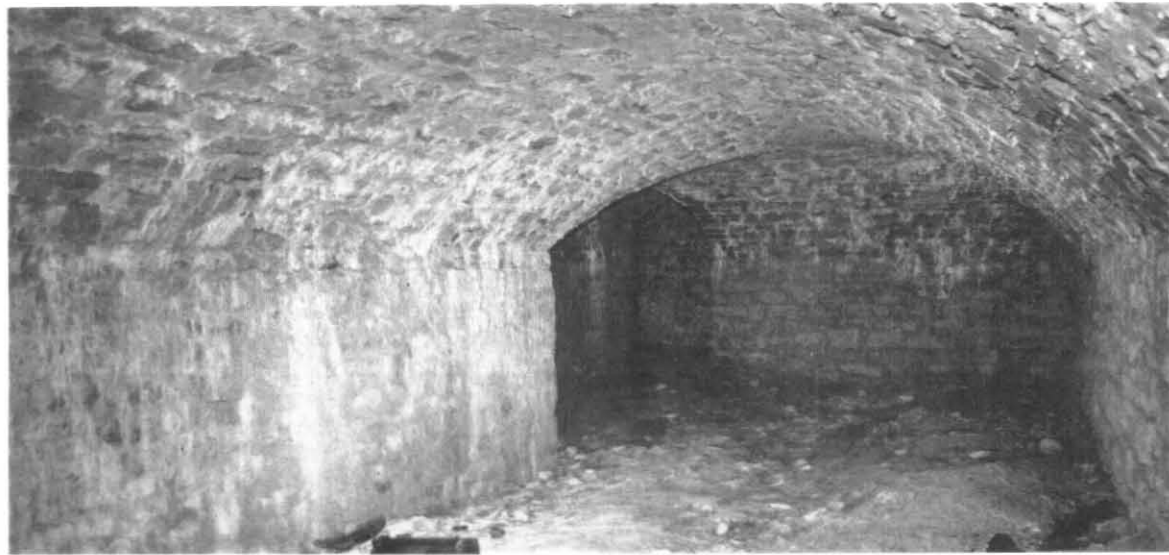
March 1992. C&V basement North side of main vaults, looking West
